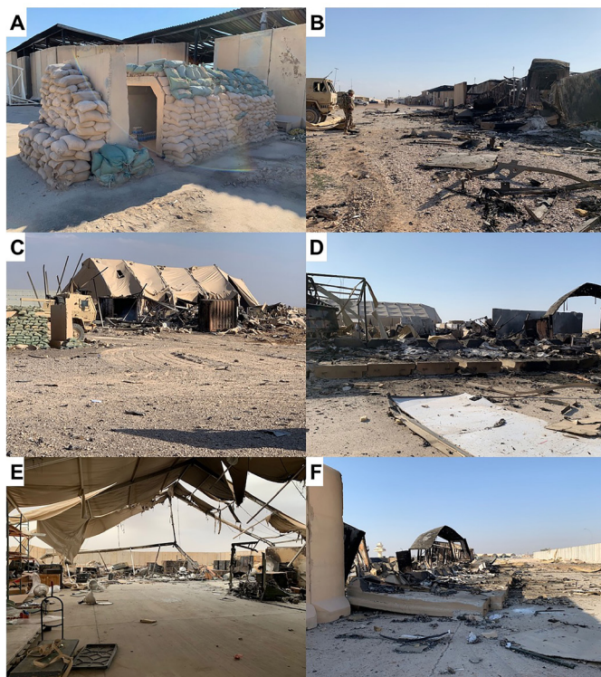
Figure 1 Images of the aftermath following the 8 January 2020 theatre ballistic missile attack on Al Asad Air Base, Iraq. (A) Most soldiers sought cover in C-shaped concrete bunkers. Image of bunker before the attack. (B–F) Images of Al Asad Air Base after the attack. All images courtesy of Alan Johnson.
